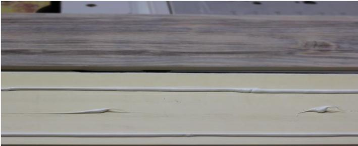
2. Apply the risers before the treads like any normal tread/riser installation.
