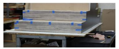
5. Install the treads following the same gluing schedule as the risers. Add one additional bead in the corner of the 90-degree angle on the back side of the bull nosing as shown below.
