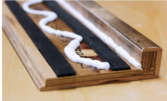
Set in place and allow five minutes to set properly. Do not walk on any newly installed stair nosing for twenty-four hours. Anticipate a yield of two 8' long stair nosings per tube of adhesive. Marking the stair nosing for one day with tape and a sign stating "DO NOT WALK ON NOSING" is suggested.
